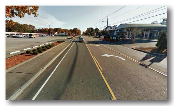
Route 109 in Medway Two-lane, two-way roadway with a two-way left-turn lane and sidewalks
