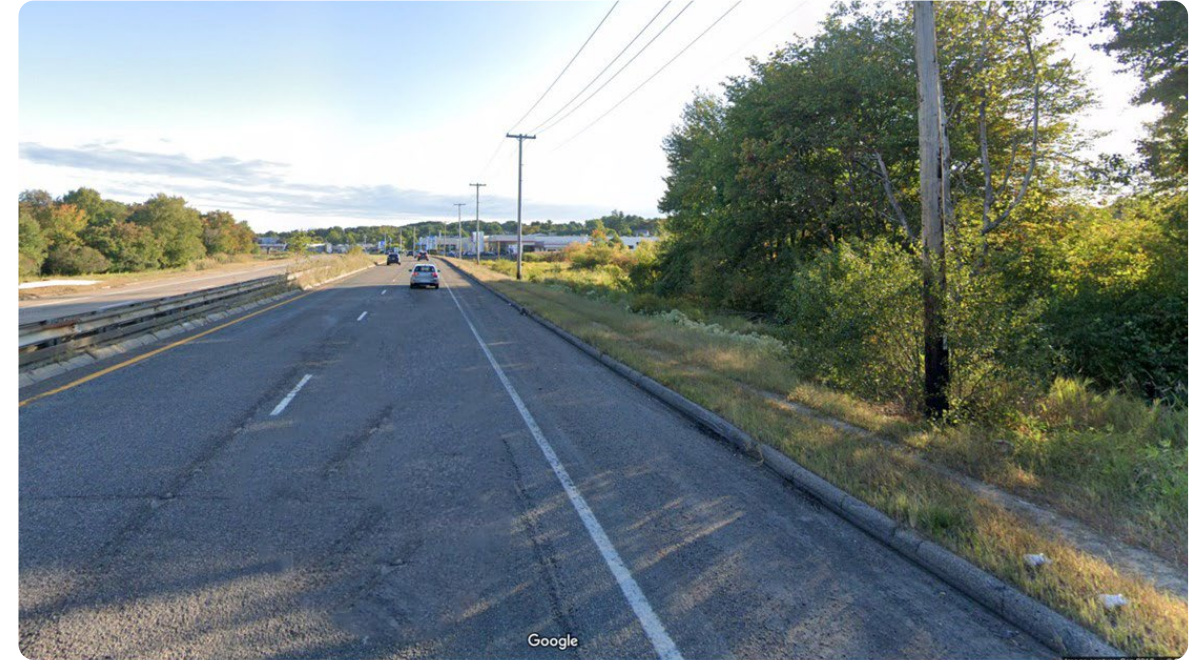
Gap in sidewalk network near Everett Street
