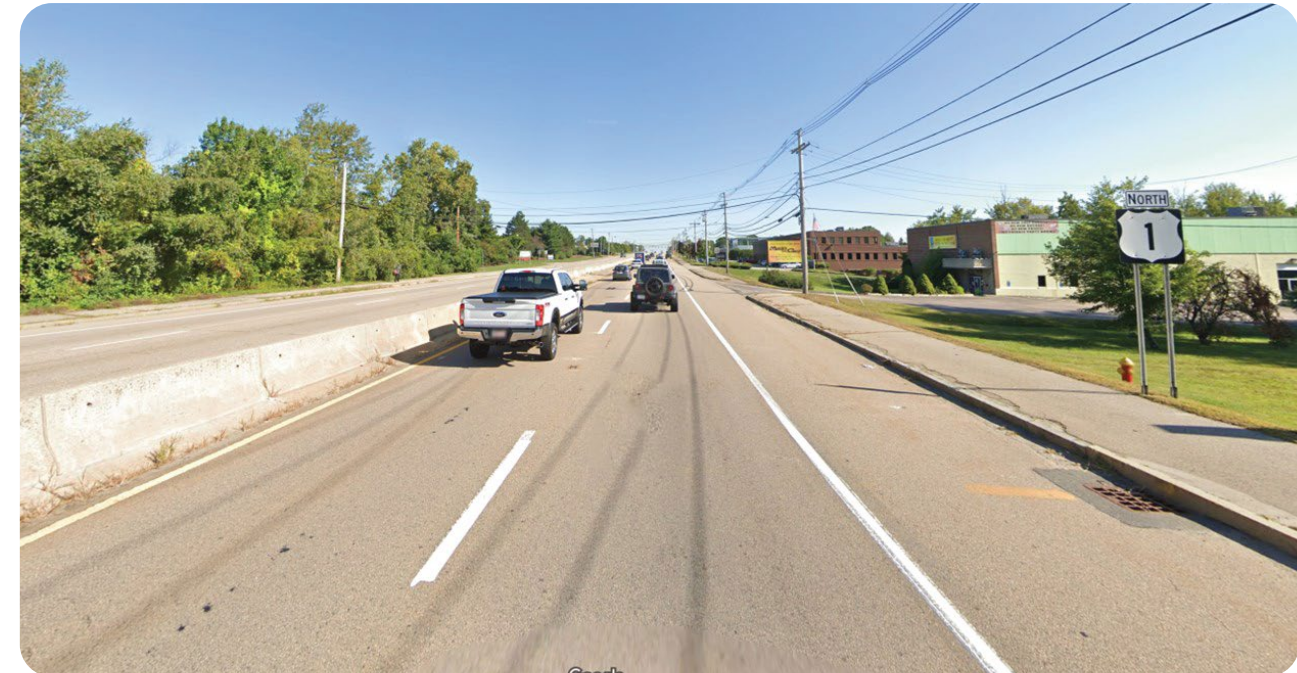
No buffer and protection for people biking on the shoulder on Route 1
