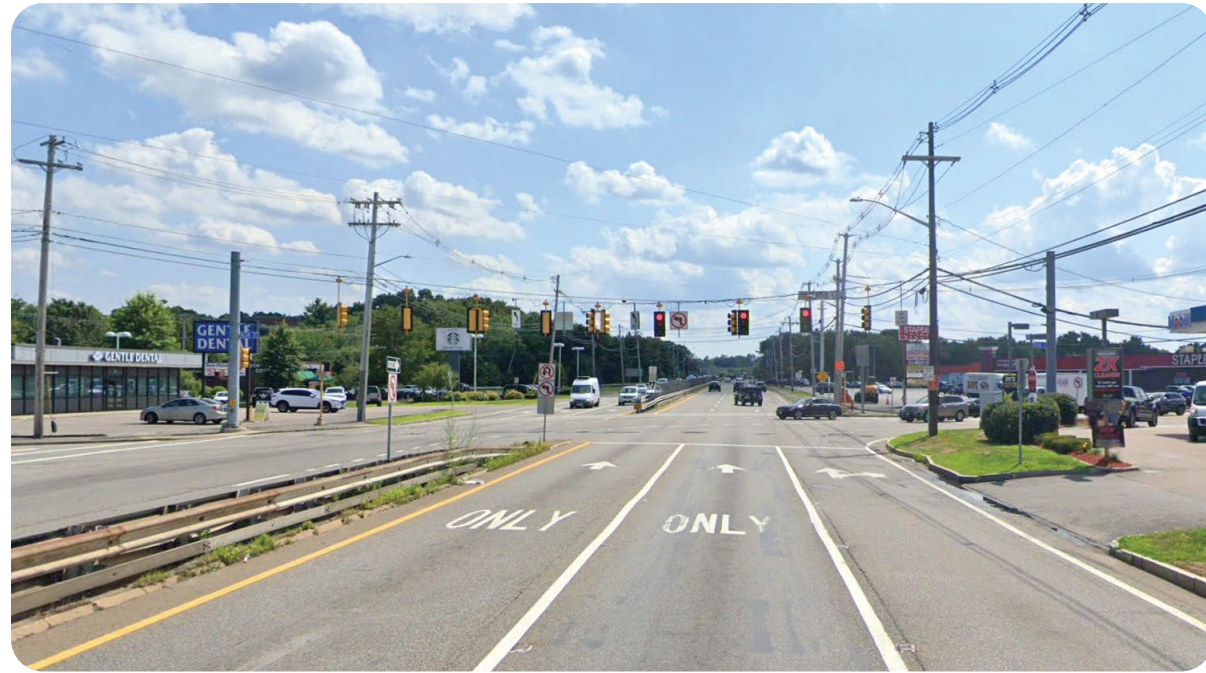
Shoulders on Route 1 end at signalized intersection because of turn lanes
