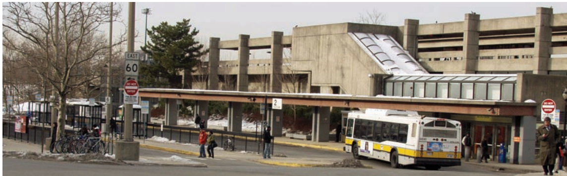
The Malden Center MBTA station is a key transit hub within the Route 60 study area providing connections to commuter rail, subway, and bus service. The MPO studied ways to improve bus service reliability along this corridor.
