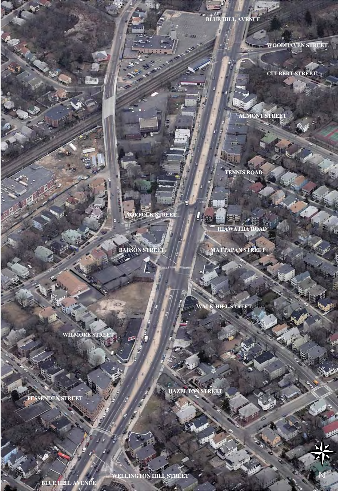
Figure B-23: Wellington Hill Street to Woodhaven Street via Blue Hill Avenue (South View)
