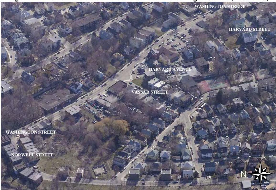
Figure B-9: Norwell Street to Harvard Street via Washington Street (East View)
