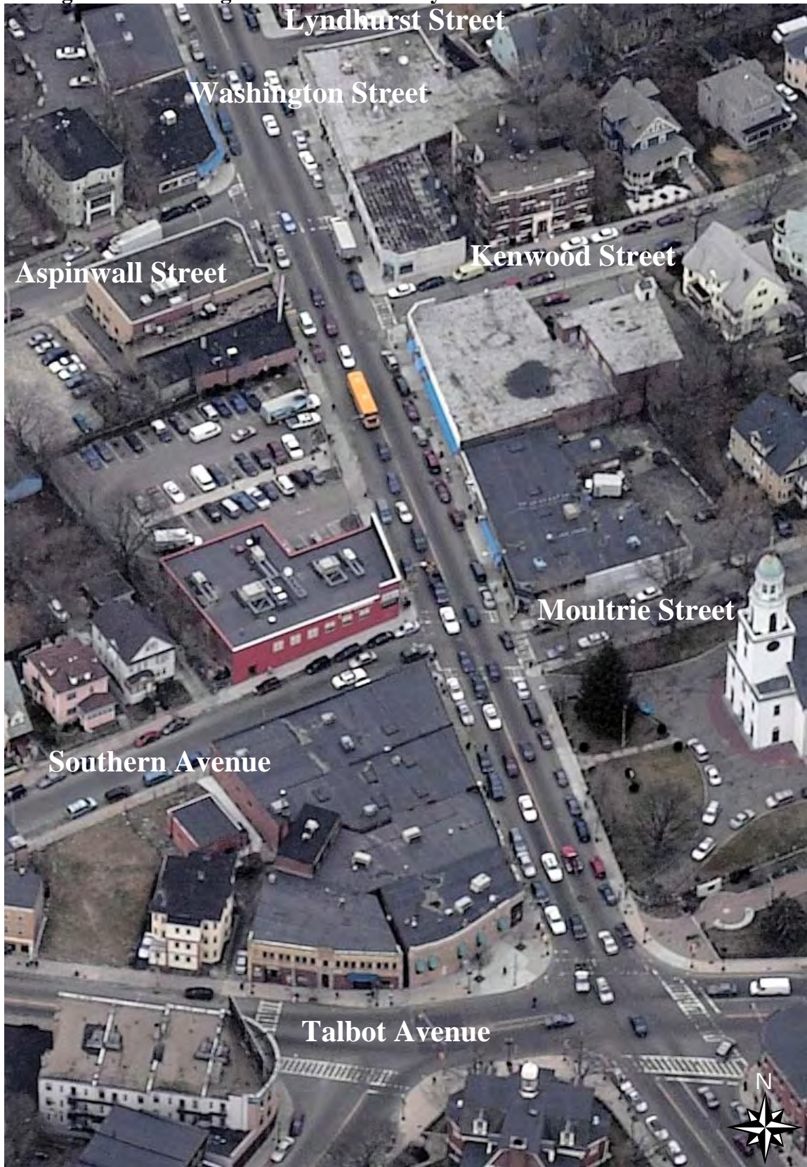
Figure 64: Washington Street between Lyndhurst Street and Talbot Avenue
