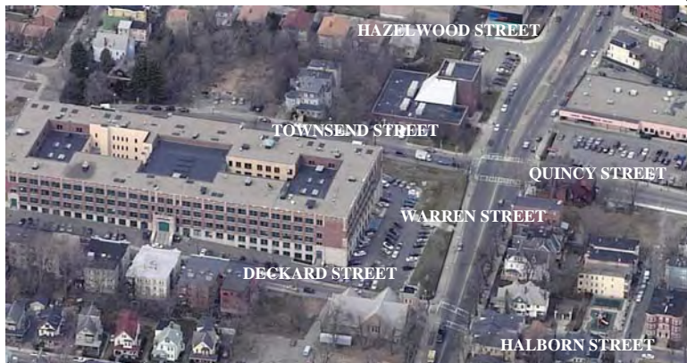
Figure B-3: Hazelwood Street to Deckard Street via Warren Street (North View)
