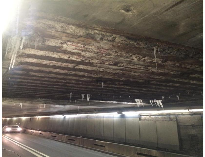
Delaminated Concrete & Corroded Ceiling Beams
