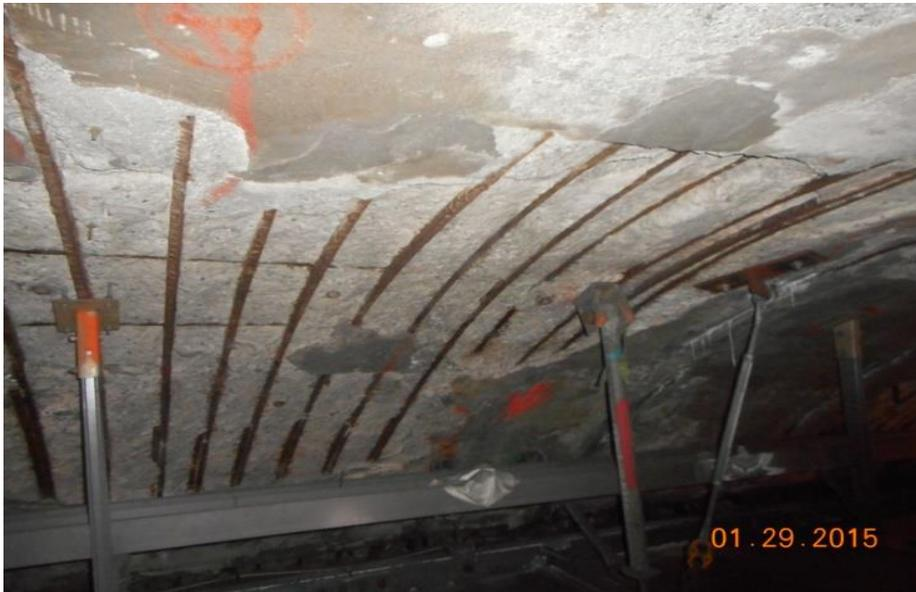
Delamination/Exposed Corroded Rebar in Ceiling
