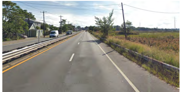
Route 1A north of Revere Street
