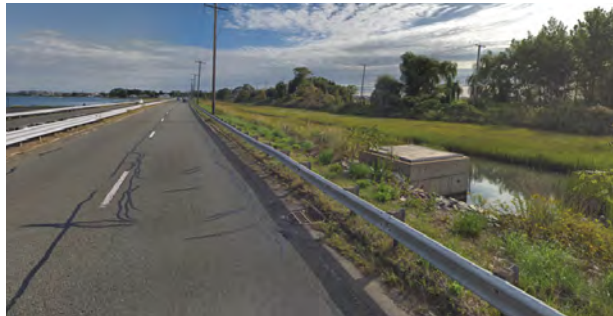
Route 1A at the Marina (east side of the roadway)
