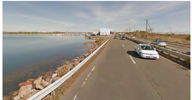
Route 1A south of the Marina
