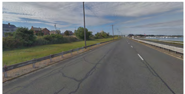
Route 1A near Mills Avenue (east side of the roadway)
