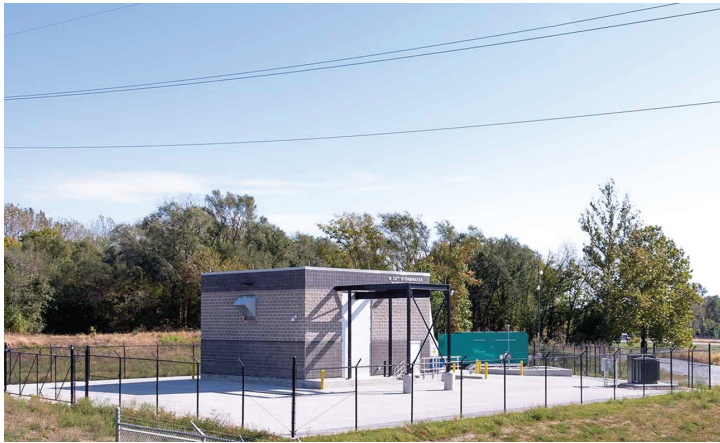
Stormwater pump station
