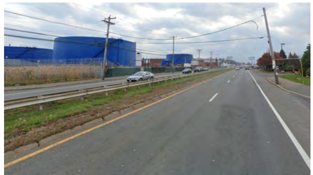
Route 1A at the oil and gas storage tanks near the Boston city line
