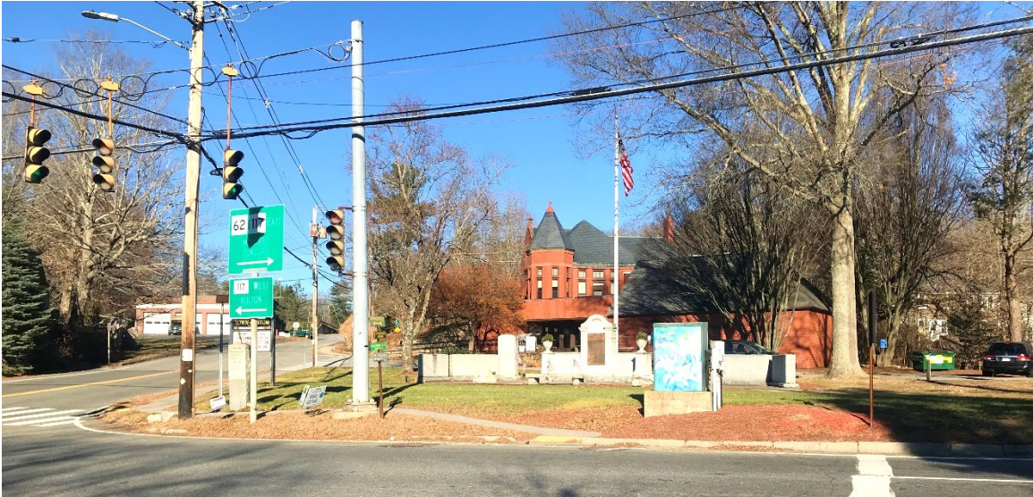
Figure 4 View across Great Road (Routes 117 and 62) of Northeast Intersection Corner
