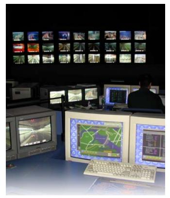
and controlling communications, monitoring carbon monoxide (CO) levels, controlling ventilation for the tunnels mentioned above, working with the Massachusetts State Police E-4 Units on enforcement actions, such as vehicle towing and providing digital videos for motor vehicle accident investigations, and working with the Boston Fire Department on fire prevention and firefighting issues and activities.
