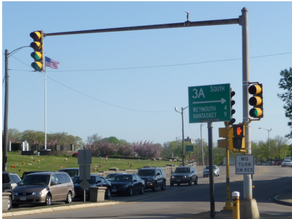
FIGURE 4 A Signal Head Mounted on a Mast Arm Pole: Southern Artery at Sea Street/Coddington Street
